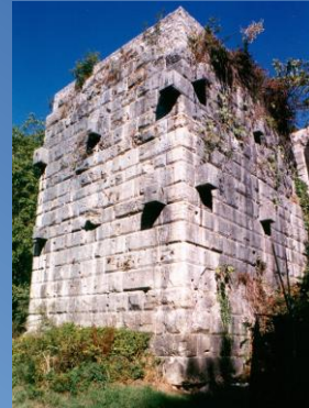
Square units work
